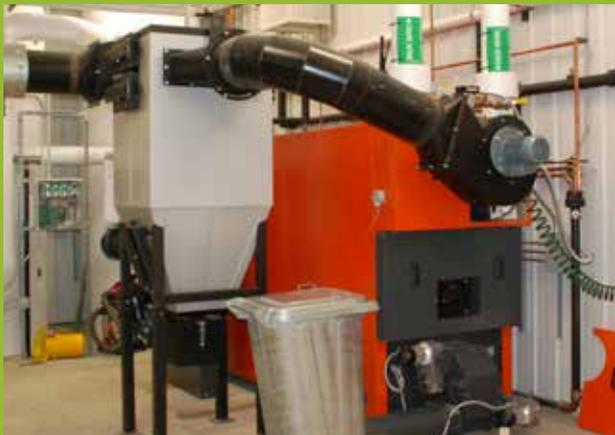
Starting in March 2017, homegrown perennial grasses will replace propane as the primary heat source for the Illinois Energy Farm's main research greenhouse. A state-of-the-art Heizomat biomass boiler produced in Germany will turn biomass into hot water distributed across the research complex as the primary energy source for heating.
