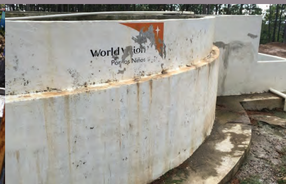
The deteriorating Las Mesas water structure: a relic of fly-by development. Credit: Taylor Jennings
